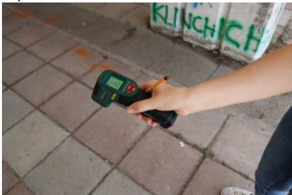
paving surface under the bridge/passage: 25,7 °C
